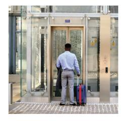
A hydraulic transit elevator is primarily used in low-rise applications. Typically serving 2 – 5 floors, their height can occasionally top 50 feet, especially in roped hydraulic configurations.
